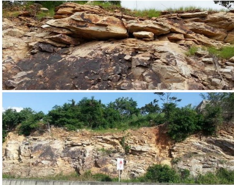
Figure 5. Slope face of RS11
